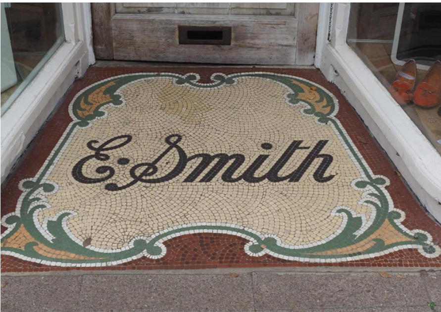
'Original Shop Front'
